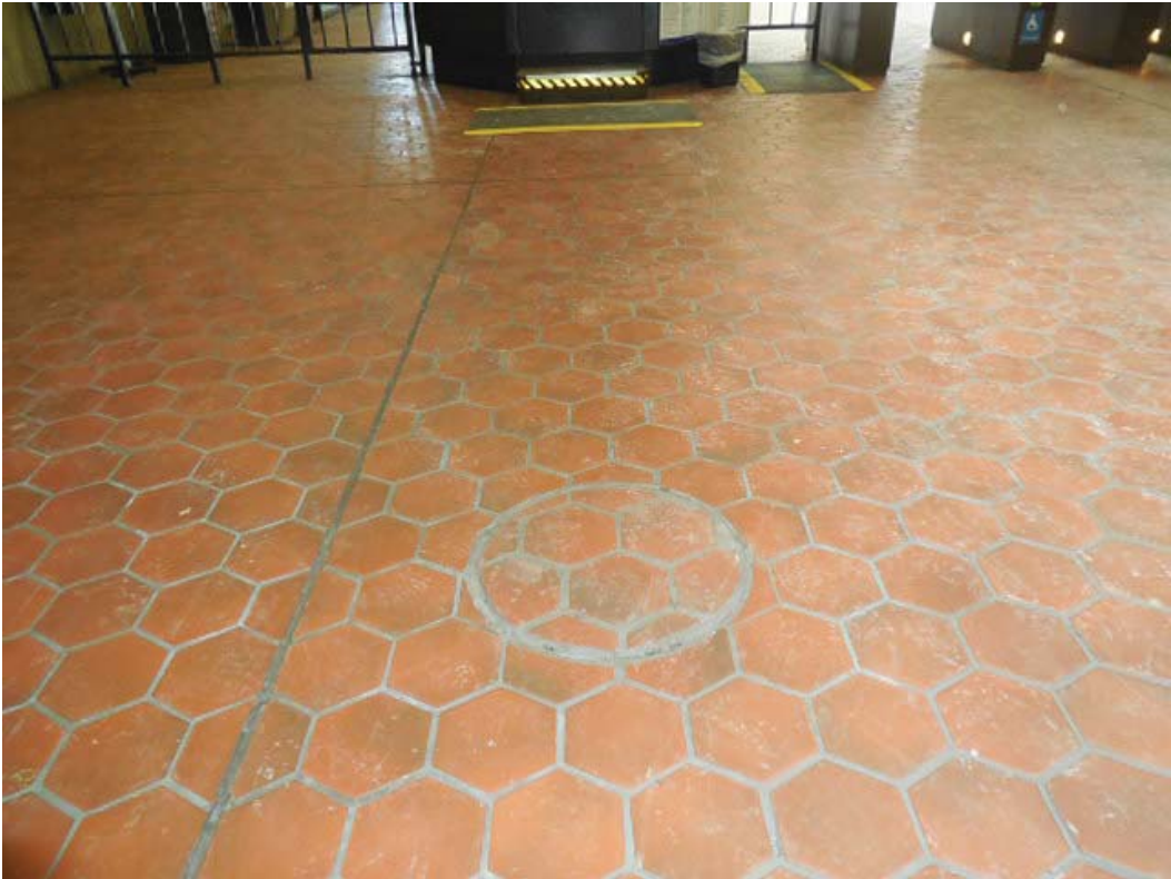
Picture 3: K05 East Falls Church – Manhole in mezzanine
