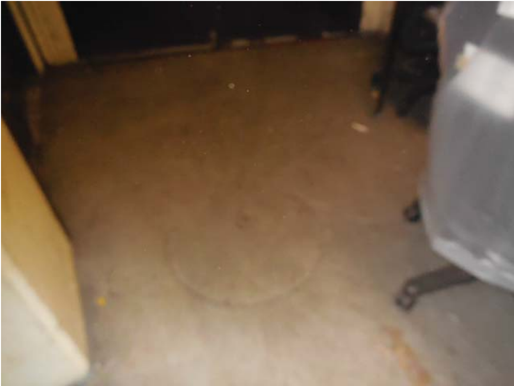
Picture 3: K02 Clarendon – Manhole in maintenance area off of mezzanine
