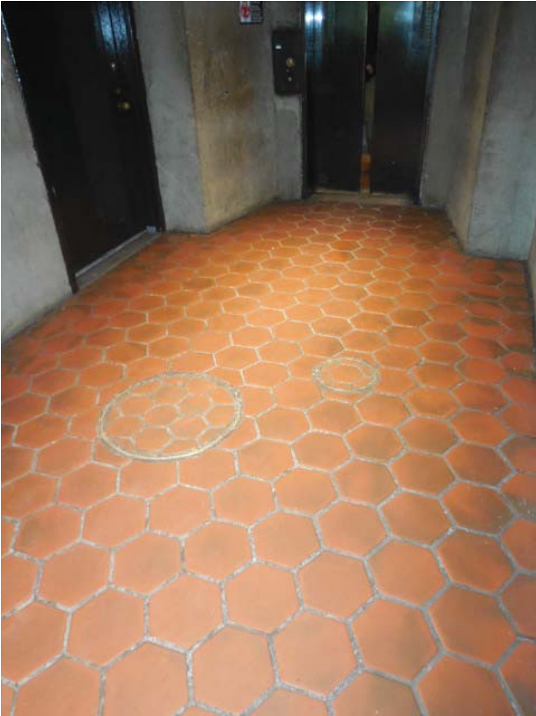
Picture 1: K01 Court House – Manhole & handhole in mezzanine
