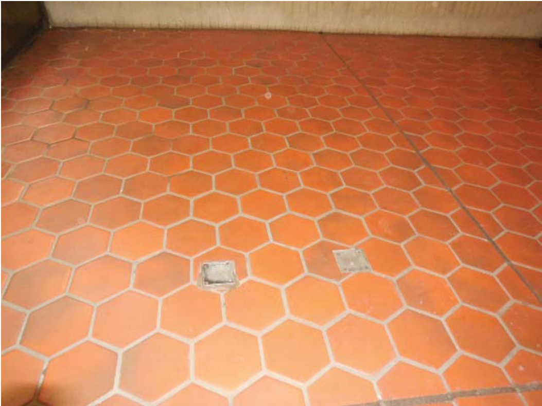
Pictures 1&2: K05 East Falls Church – Handholes in mezzanine
