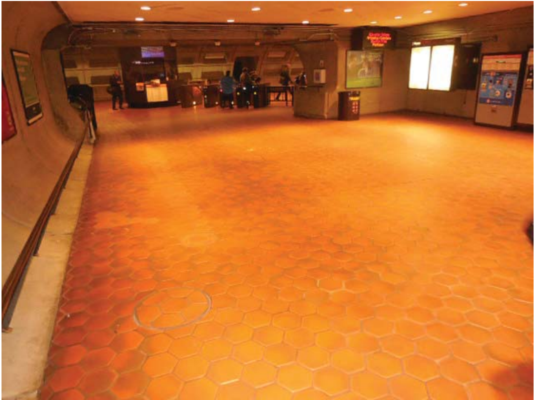
Pictures 1&2: K03 Virginia Square-GMU – Handholes & manholes in mezzanine
