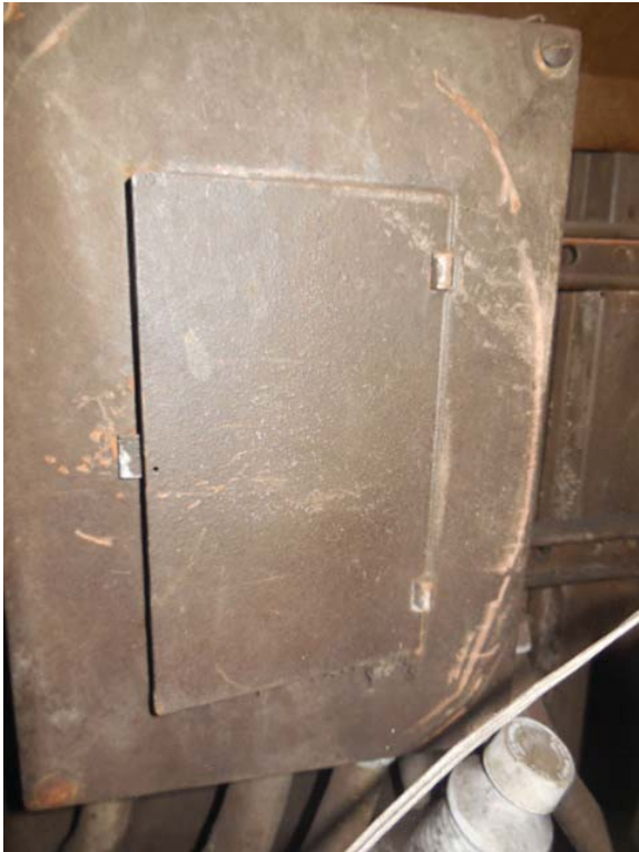
Pictures 3&4: K03 Virginia Square-GMU – Emergency Panel KE in Kiosk
