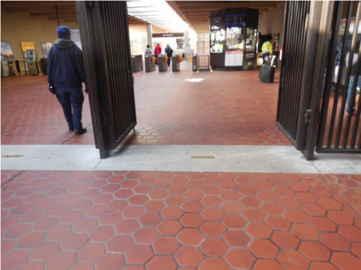
Picture 1: K08 Vienna – Handholes in Mezzanine
