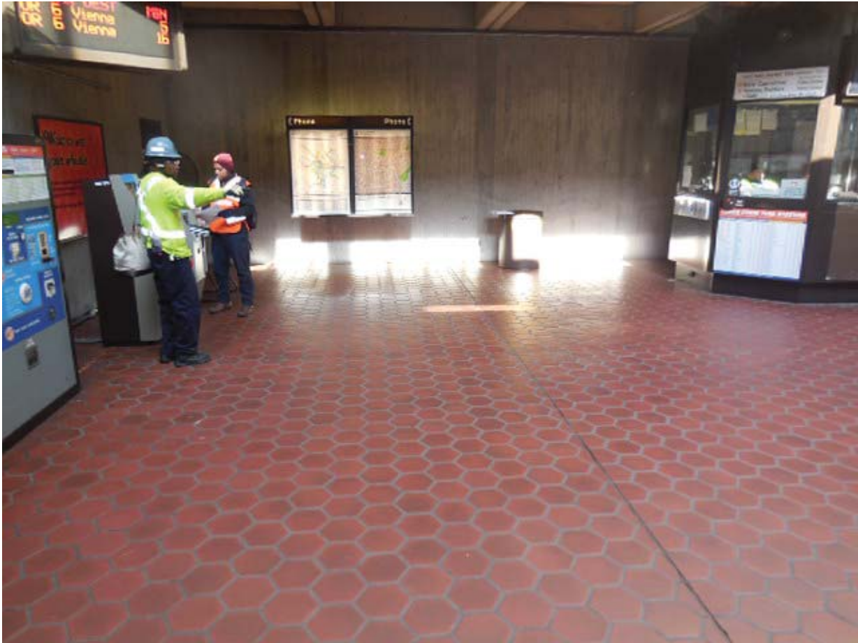
Picture 2: K07 Dunn Loring – Handholes in Mezzanine
