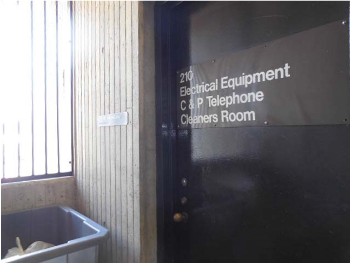
Picture 3: K06 West Falls Church – Room 210 in Mezzanine which leads to Room 212 electrical room
