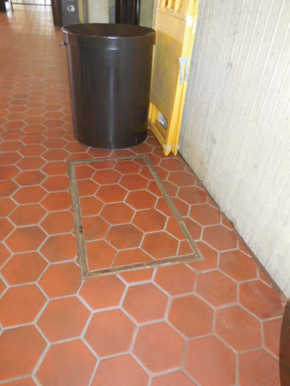
Picture 2: K06 West Falls Church – Unassociated access hatch in Mezzanine
